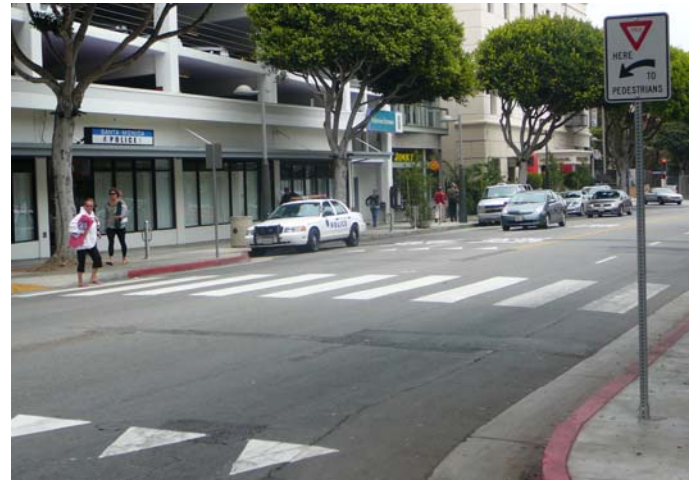
Triangular yield markings and accompanying signage at an unsignalized crosswalk
