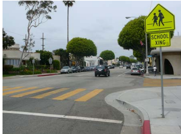
Intersection Curb Extension with Dual Curb Ramps
