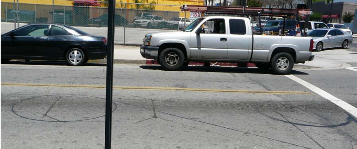
Existing vehicle detection on Maple Street at Central Avenue (loops in pavement)
