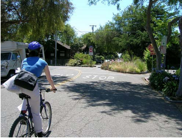
A landscaped diverter provides a gap for bicyclists to continue through the intersection while motorists are forced to turn.
