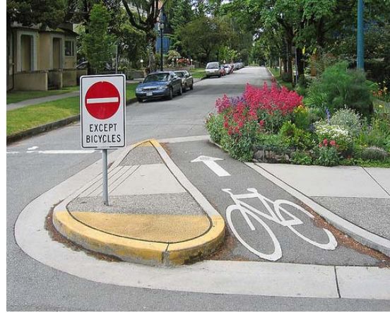
A partial closure allows for two-way bicycle traffic and one-way motor vehicle traffic
