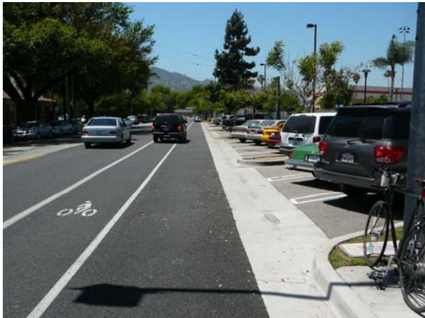
North side bike lane west of Pacific Avenue
