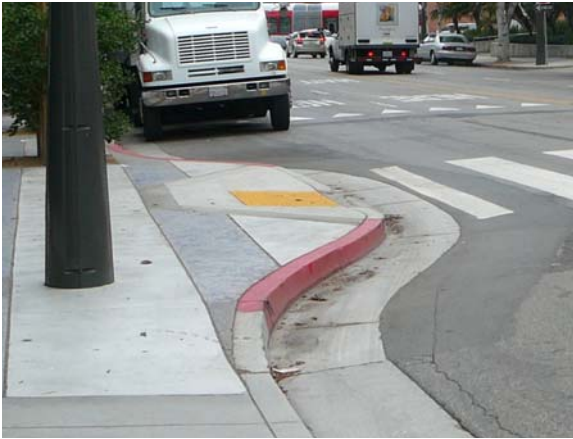
Midblock Curb Extension
